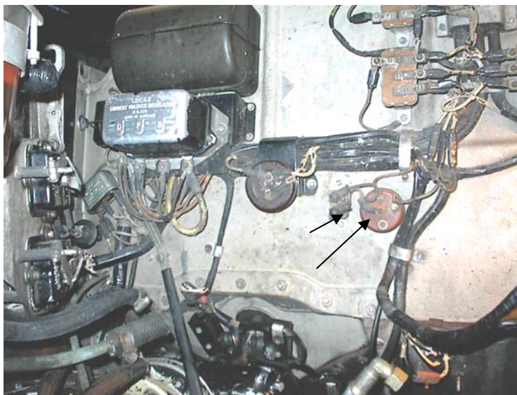
As fitted to the first V8's. The Otter switch is on the left
