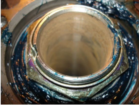
The new nut is staked. Beneath it is the keyed thrust washer
